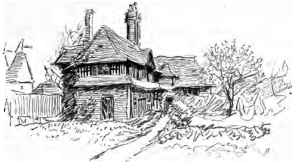
Half-timbered House, Rawlinson Farm, Rolwenden.
